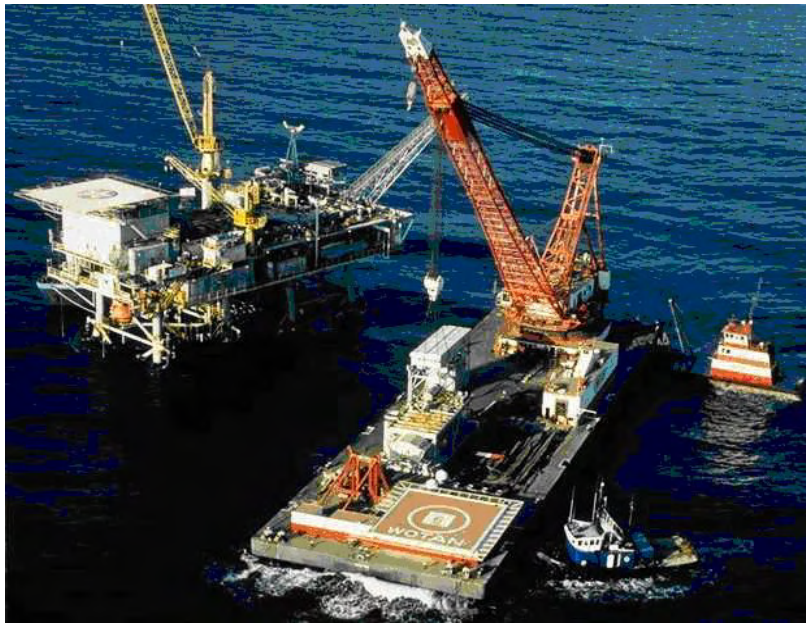
Figure 8 - Manson Construction 600-ton Derrick Barge WOTAN operating offshore
